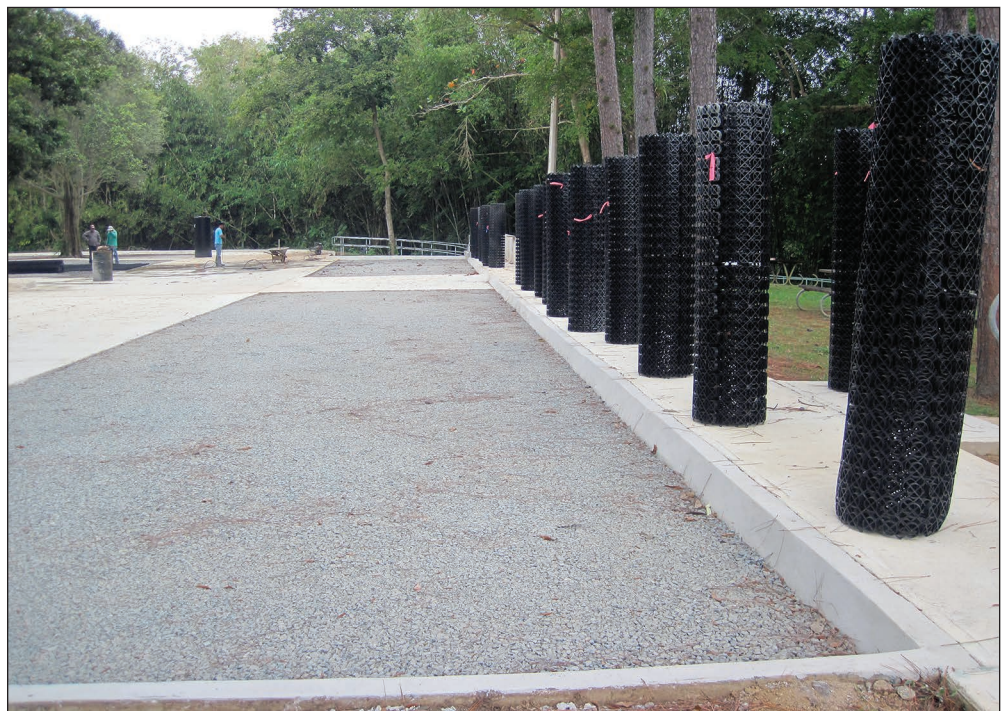
Figure 33—The Green Parking Lot has several layers of materials. Black plastic rings seen on the sidewalk were added to these layers to provide strength to the system.
