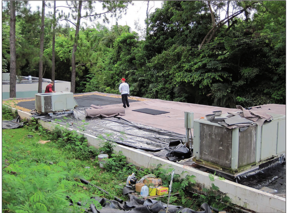
Figure 19—Layering of materials over cool roofs in preparation for the green roof of the Geographic Information System and Remote Sensing Laboratory.
