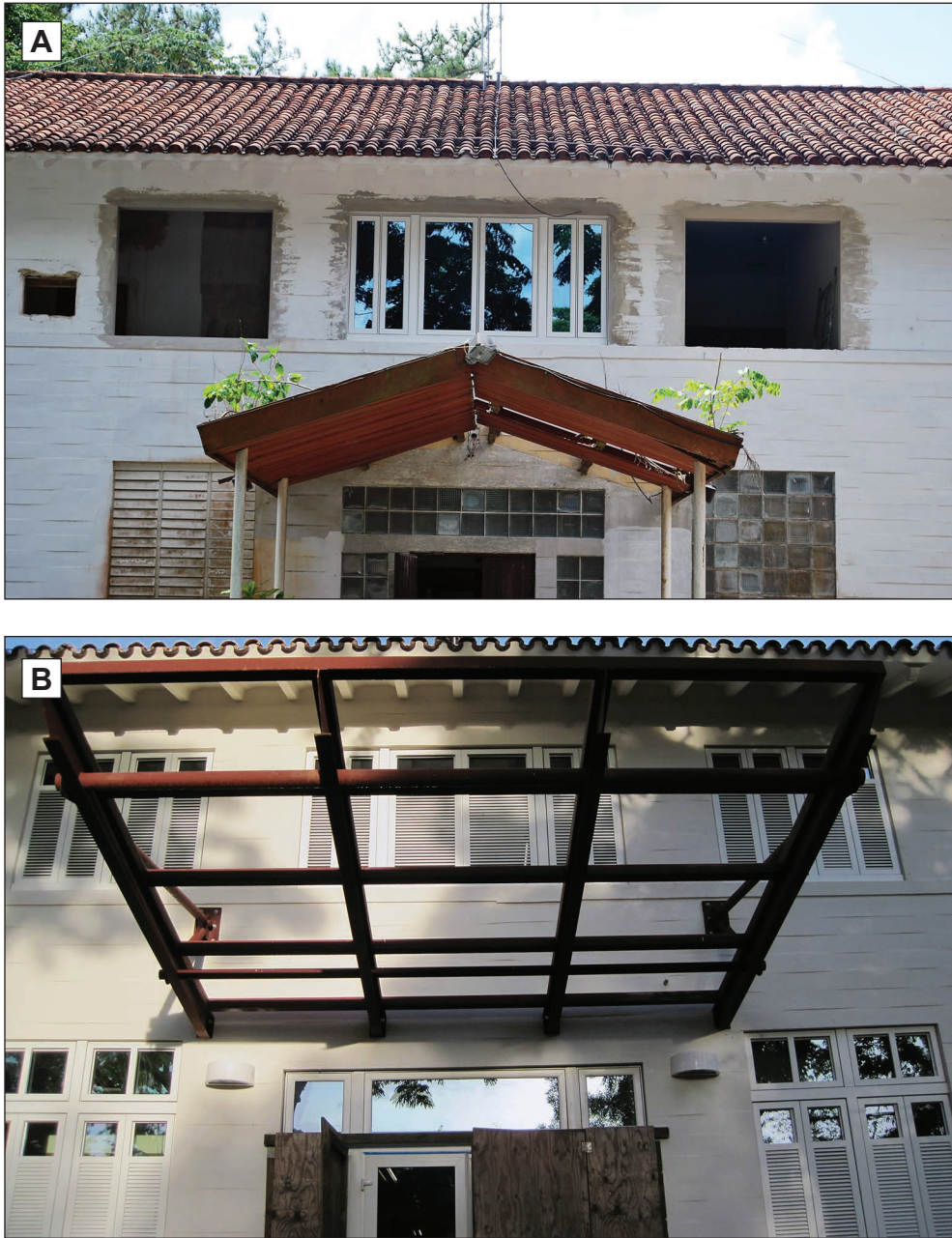
Figure 32—The Institute building had an entrance portal on the west end facing the parking lot (a), which was not part of the original building design. We retained the function of this portal with the installation of a new structure (b), which has not been painted as designed, owing to budget limitations.
