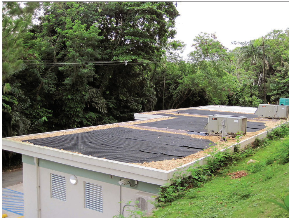
Figure 13—Preparation of the green roof of the Geographic Information System and Remote Sensing Laboratory for planting of green vegetative material.
