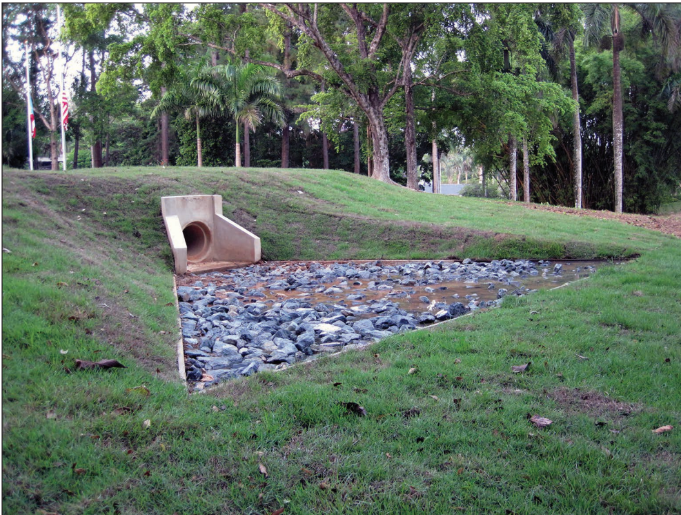
Figure 22—Outlet for the hydrologic system of the Green Parking Lot. Rocks dissipate the energy of outflowing waters before they flow downslope through the lawn, which acts as a green swale that absorbs and evaporates water.
