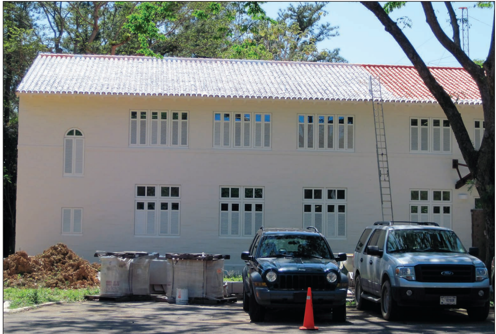
Figure 11—Restoration of the roof tiles of the Institute building. Notice also the new windows.
