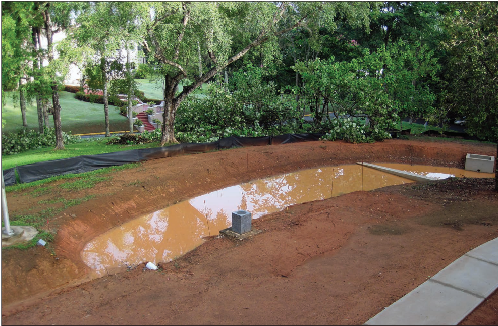
Figure 21—Construction of the concrete sidewalks, open water canals, and detention pond in front of the Institute Building. The system outlet is the concrete box on the far right. The muddiness of the water is due to construction work. The marble cube in the center is a calibrated monument for the Geographic Position System Coordinates of this location. The official name for this cube is 100 Year Commemorative Monument and High Accuracy Geodetic Control Mark.
