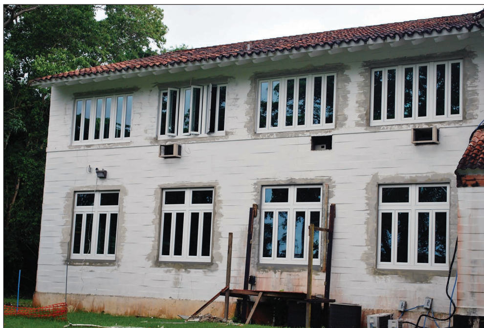
Figure 27—Installation of new windows at the Institute building.
