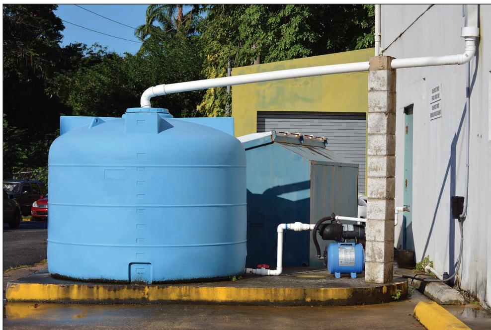
Figure 20—The roof rainwater collecting system in back of the Frank H. Wadsworth Library. Shown are the drainage pipes from the roof to the blue cistern, pump used to return water to the roof during draught conditions, and blue cistern where water is stored.
