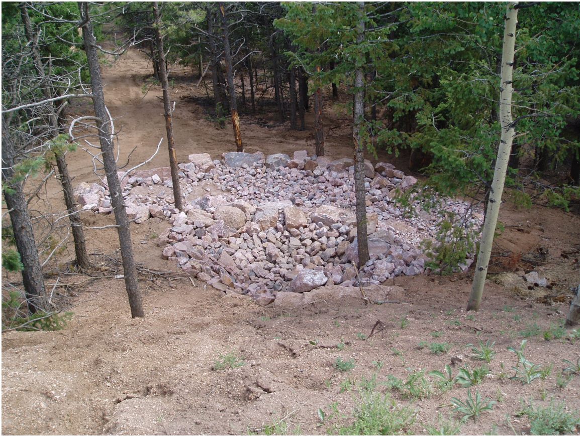
Figure 12. Reconstructed velocity dissipater above 175CC August 3, 2004.
