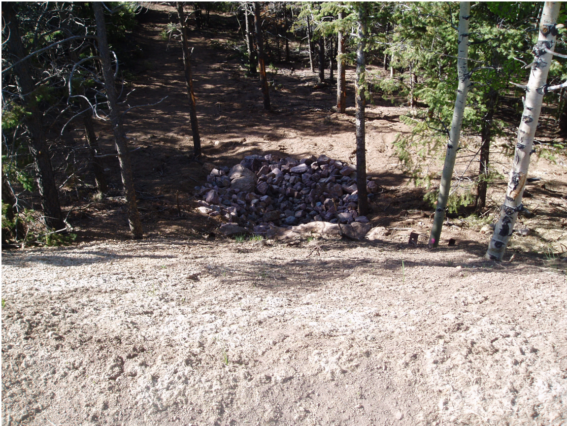
Figure 11. Velocity dissipator near site 007FS and above 175CC, June 2, 2004.
