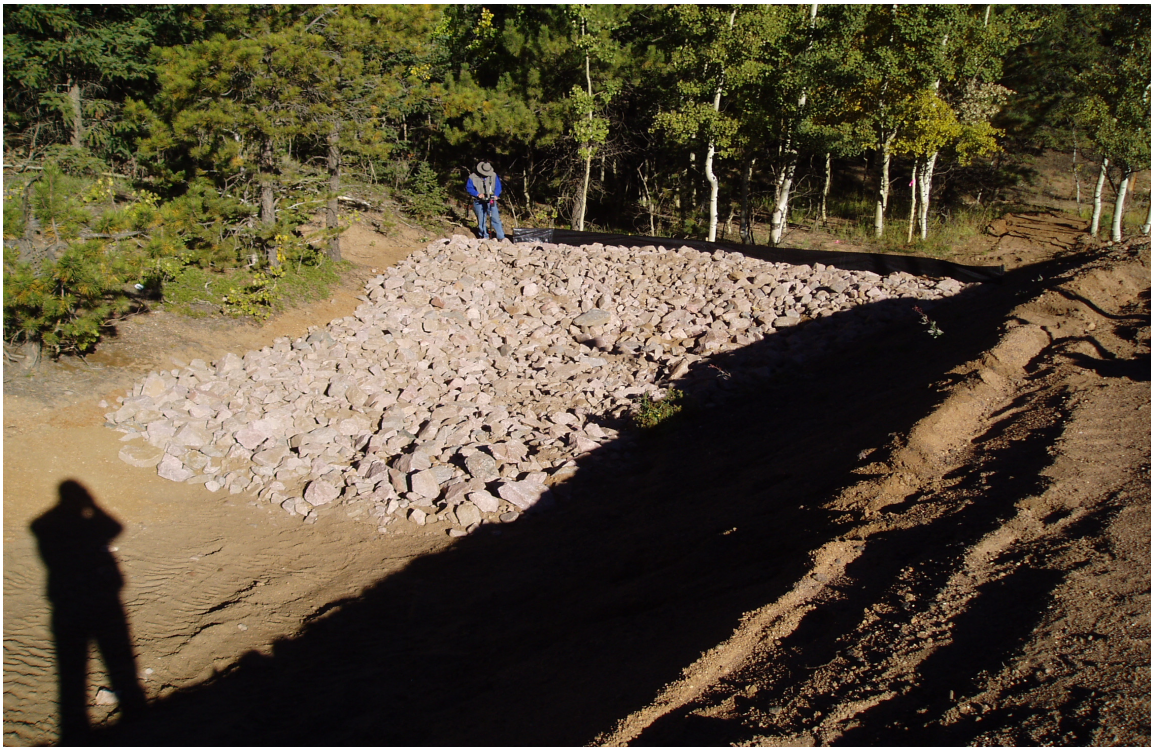
Figure 10. Rock apron site 163RA September 2003.
