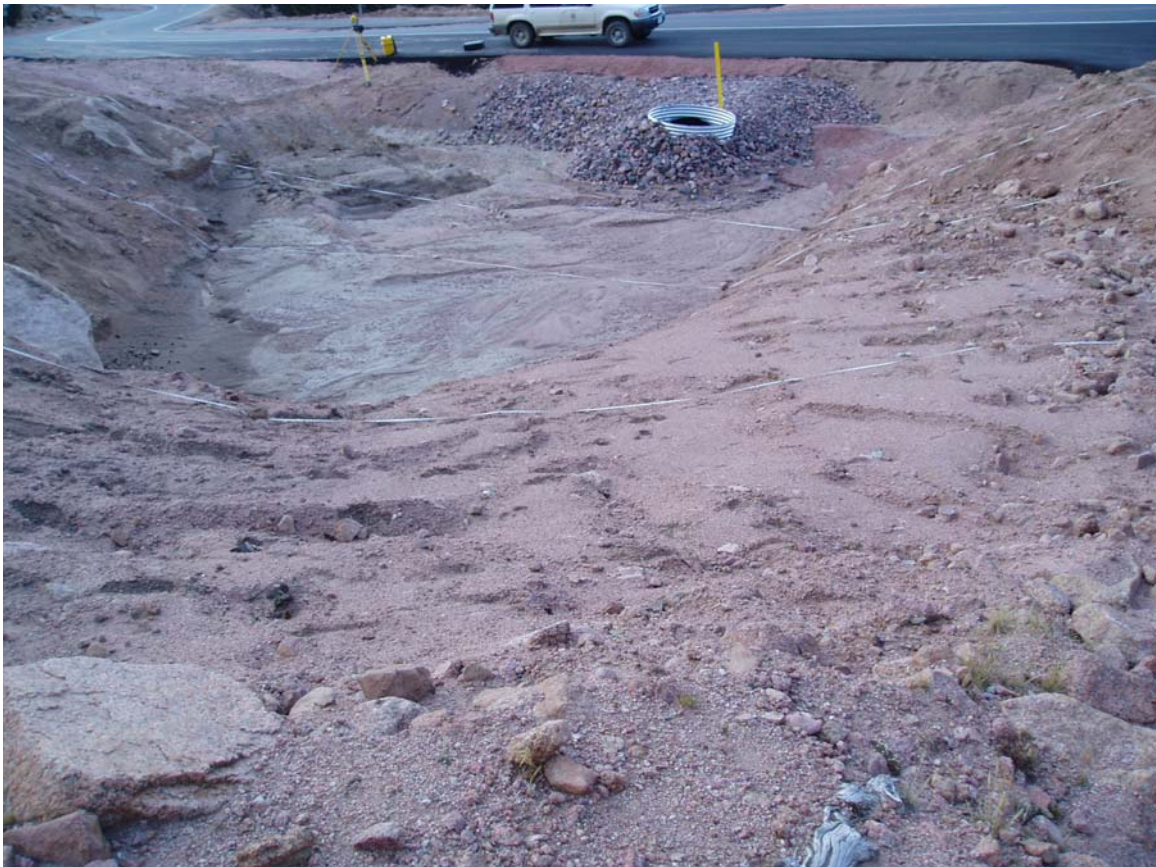
Figure 9. Sediment pond 237RW below Ski Creek diversion wall.
