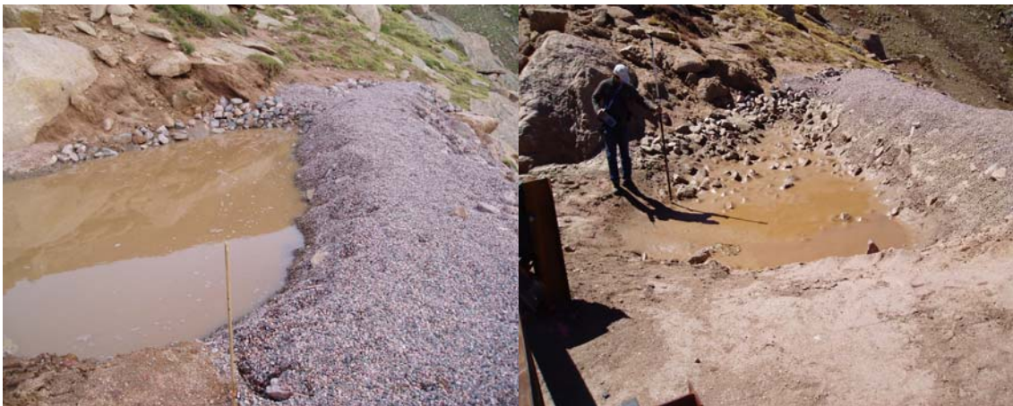
Figure 8. Storm runoff in rock weir 236RW on August 20 th (left) is still present on September 1, 2005 (right).
