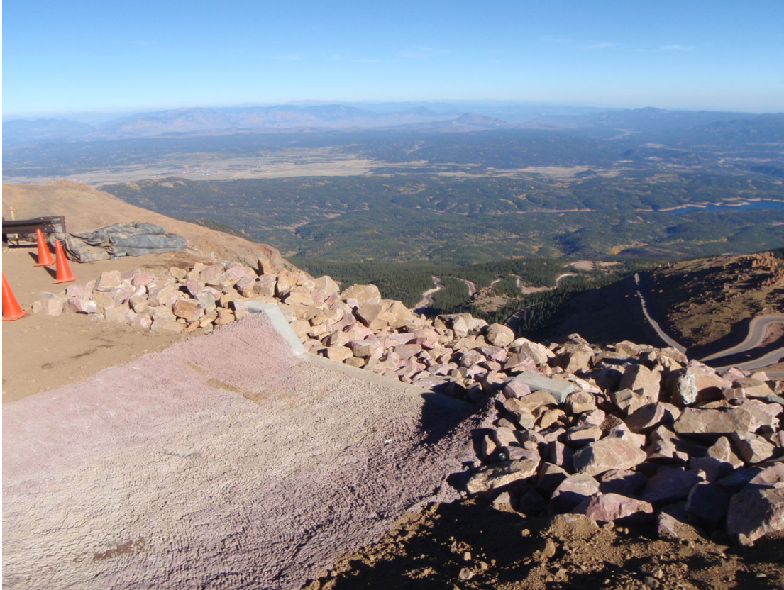
Figure 4. Rock weir 243RW was removed and replaced with cutoff wall with riprap apron below Pikes Peak, 2012.
