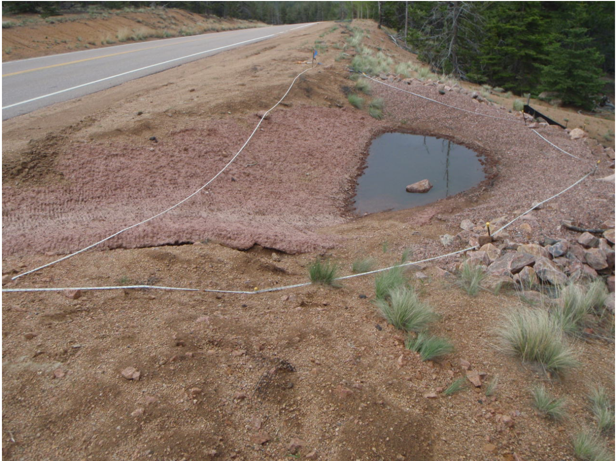
Figure 9. Rock weir 176RW lined with shotcrete and filled with standing water. The high flow is causing the shotcrete to be undercut, Pikes Peak 2014.
