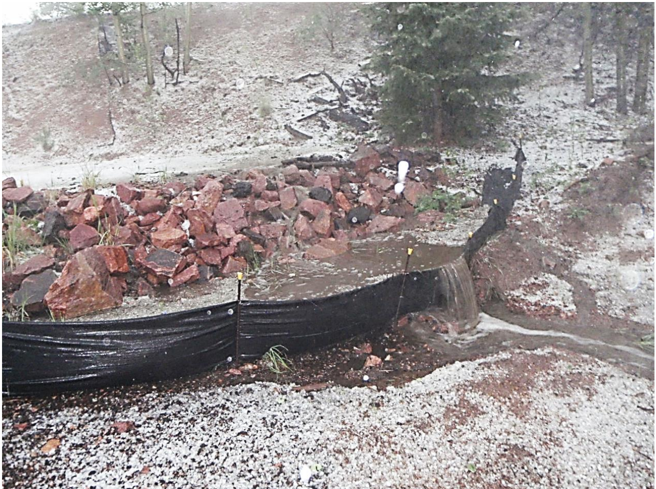
Figure 8. Rock weir 202RW overtopping during storm event on July 8, Pikes Peak 2014.
