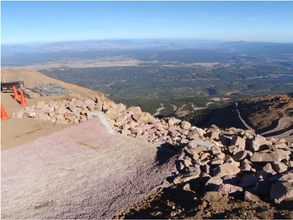
Figure 7. Rock weir 243RW was removed and replaced with cutoff wall with riprap apron below, Pikes Peak 2012.
