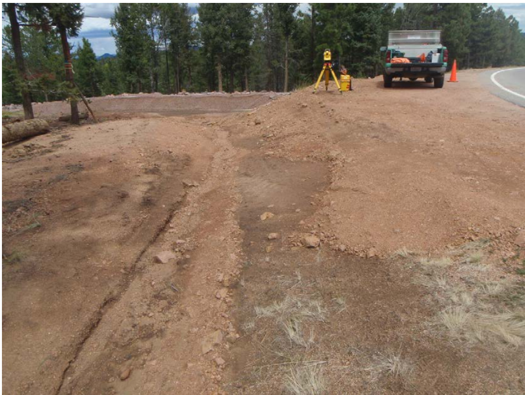
Figure 1. Rock weir 009RA with temporary access road crossing contributing ditch (top) and drainage ditch after removal of material at the end of the field season (bottom), Pikes Peak 2014.
