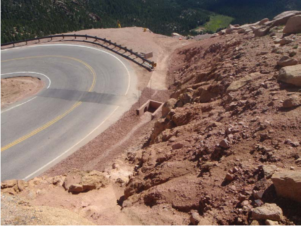
Figure 6. Pipe back under the highway above rock weir 234RW which diverts water entering Severy Creek to a shotcrete ditch above sediment pond 237RW which flows into Ski Creek, Pikes Peak 2014.
