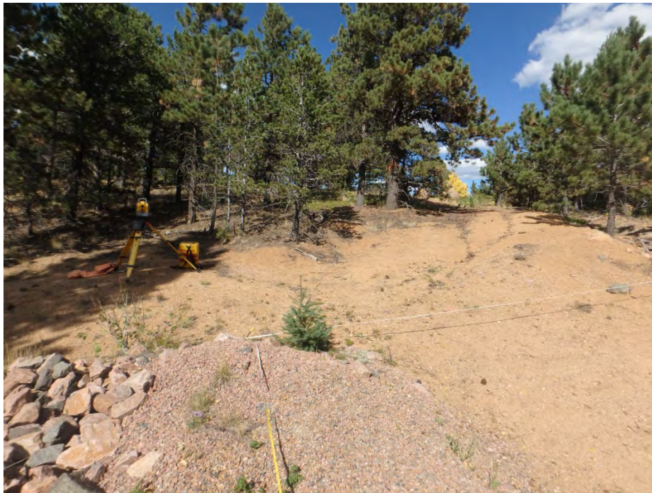
Figure 1. Rock weir 153RW showing bare apron above rock weir that could be aggravated if disturbed or stabilized, Pikes Peak 2015.
