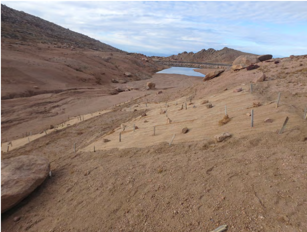
Figure 3. RMFI planted native seeds and installed erosion control fabric on the hill slope along the highway drainage flowing into sediment pond 258RW.
