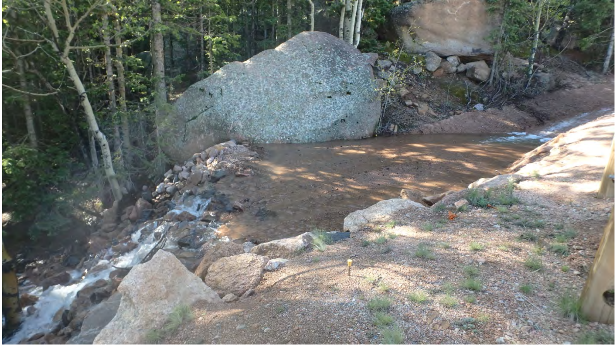
Figure 8. Rock weir 252RW filled with sediment and overtopping during spring runoff, Pikes Peak June 16, 2015.
