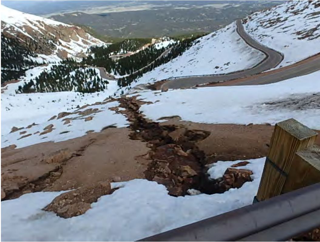
Figure 10. Water and sediment diverted away from 238RW to the fill slope below, Pikes Peak June 1, 2015.
