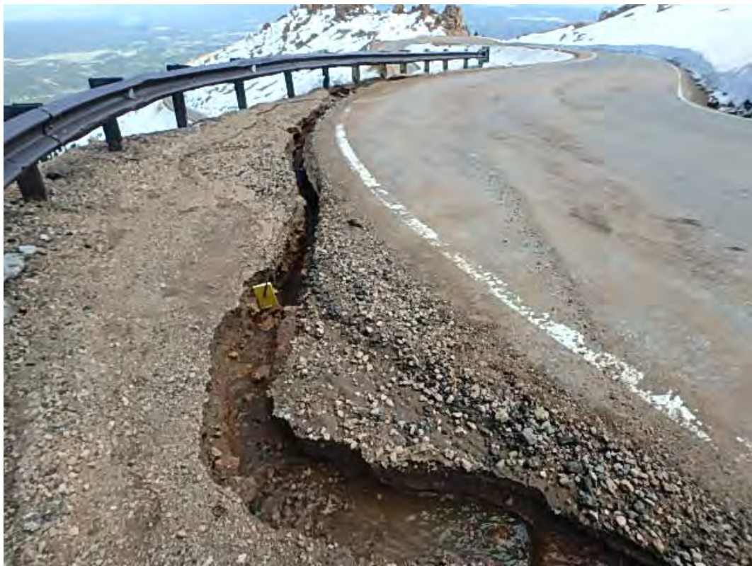
Figure 9. Ice block above 238RW (top) diverted water away from the rock weir and down the side of the highway (bottom), Pikes Peak June 1, 2015.
